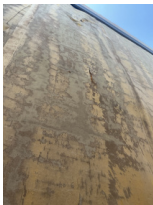
Trailer Right Side
